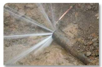
Figure 6: Underground leak running at high pressure (Ken Brothers)
