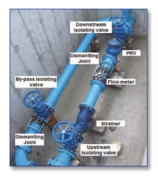
Figure 9: Typical bulk management meter in pressure reducing valve (PRV) chamber
