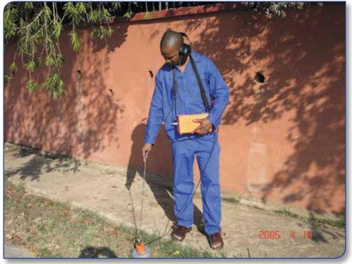
Figure 4: Leak location using sounding equipment
