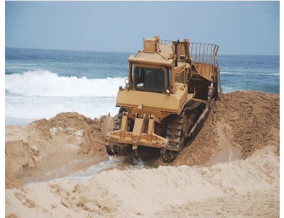
Mechanical breaching of a sandbank
