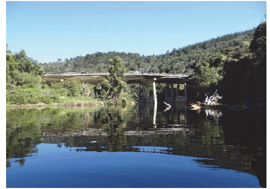
N2 bridge across the Kaaimans Estuary, Western Cape
