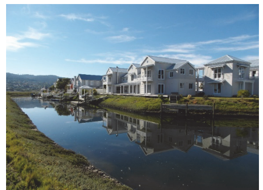
The Motherwell Canal carries stormwater run-off and sometimes raw sewage into the Swartkops Estuary, Port Elizabeth
