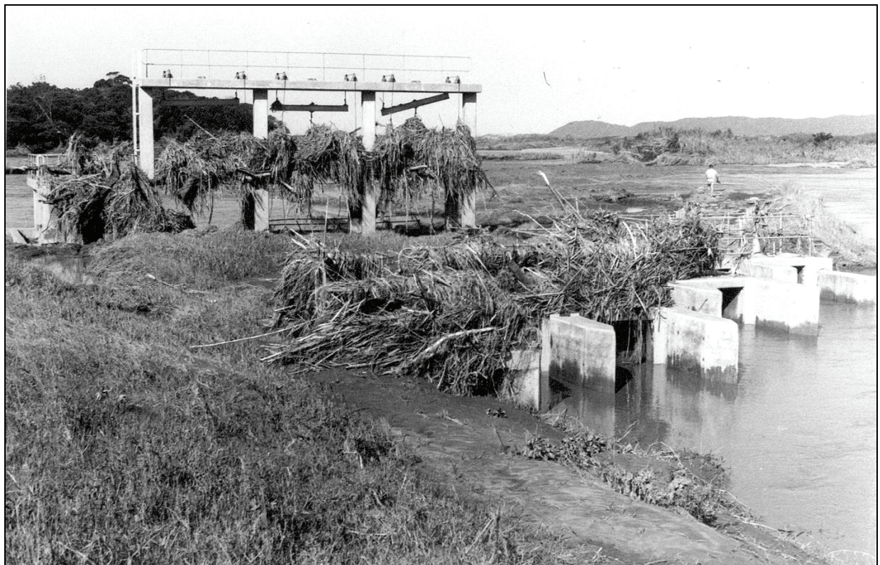
Figure 14. The Link Canal was damaged during the Domoina Flood. This photograph shows flood debris caught in the superstructure of the Intake Works (photograph: R. Taylor).
