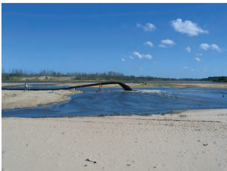
Figure 7. Maintenance dredging at the St Lucia mouth.
