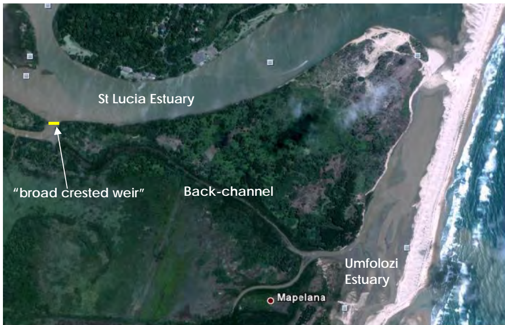
Figure 3.14 Aerial view of the back-channel (Google Earth, 2008).
