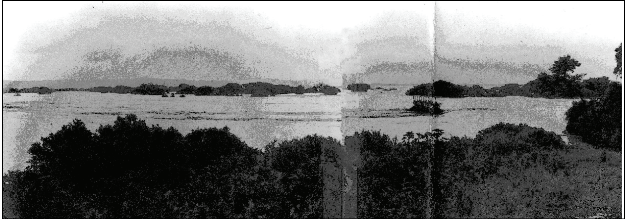
Figure 13. Domoina floodwaters filled the Mfolozi basin. In the centre-right the concrete superstructure of the Intake Works protrudes above the floodwater (photograph: R. Taylor).
