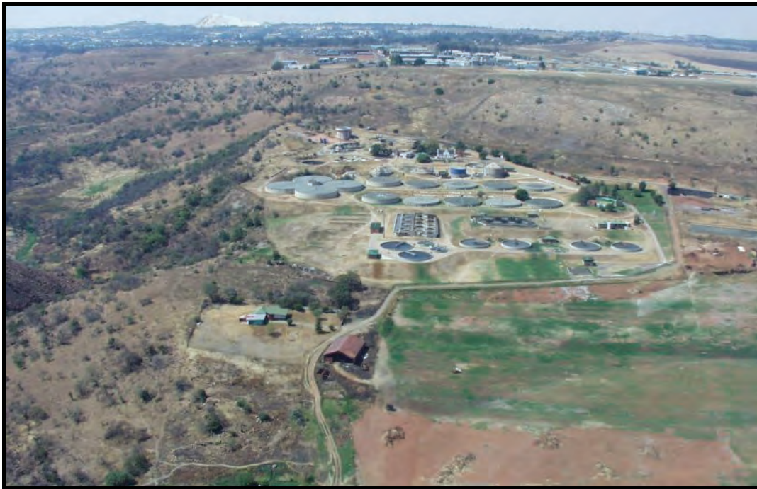
Figure 10.5: The Percy Stewart Sewage Plant of Mogale City discharges effluent into the Blougaatspruit entering the COH WHS. Behind the sewage works is the industrial area of Delporton, while still further in the background, one of the sand dumps of the gold mines is just visible on the horizon. Every-thing in the photo falls within the catchment of the Cradle. The Rietfontein Fault has created the valley along which the Blougaatspruit flows as shown in this photo to the left (east) of the sewage works (photo: W.G. Krige 05/10/2004).
