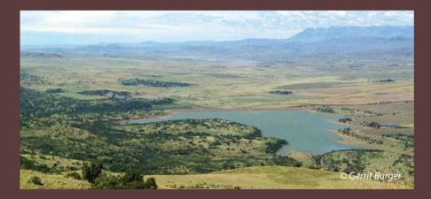
The Woodhead Dam (in the foreground) and the Spioenkop Dam (in the back) was later constructed to pump water into the Sterkfontein Dam. Whereas the prior dams fall within the catchment of the Thukela (Tugela) River draining towards the Indian Ocean, it is pumped into the Sterkfontein Dam in the Vaal River draining towards the Atlantic Ocean.
