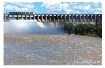
The Vaal Dam wall was initially 54.2 m at the lowest foundation and is a gravity dam comprising a concrete gravity structure with an earthfill section on the right flank. The height was increased to 60.3 m in the 1950s, and again to 63.4 m in the 1980s. The dam presently stores roughly 2 600 million cubic metres of water with an additional temporary flood safeguard just above 600 million cubic metres.
