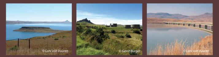
The Sterkfontein Dam stores water for release to the Vaal River. Water is sourced from the Tugela River and pumped upwards from the Woodhead Dam. The Vaal and Sterkfontein Dams are among the top five largest dams in South Africa at present.
