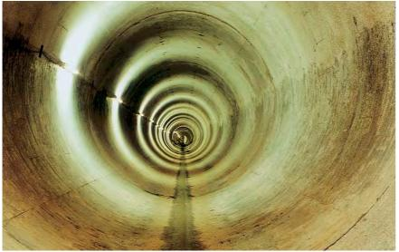
More than 80 km of tunnels were constructed to convey water from the Lesotho mountains to the Vaal River system in South Africa. The main tunnels have an internal diameter of more than 4 m.
