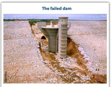
n 1993, the 38 m-high Zoeknog Dam, constructed in the Mutlumuvi River, a tributary of the Sand River, failed on first filling. The dam was constructed for the Lebowa government mainly for irrigation purposes. Investigations revealed that the dam, which had received an award from SAICE the previous year, had failed because of poor construction. Reconstructing the dam was later deemed uneconomical, and the remainder of the dam wall was demolished in 2000.
