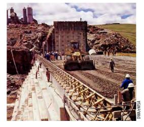
The completed mass gravity Zaaihoek Dam. Its stepped spillway – the first of its kind in South Africa, can clearly be seen.
