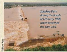
to riverbed level. Consequent investigations revealed that the breach had initially occurred at the junction between the concrete of the side channel spillway structure and the earth embankment. Once breaching started here it widened gradually. Within ten hours the dam wall failed completely, and a large quantity of eroded material was deposited immediately downstream of the dam wall.
