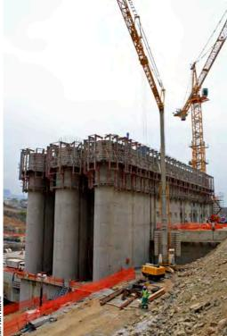
outlet structure of De Hoop Dam. The outlet works will have a maximum capacity of 20 m<sup>3</sup>/s – 15 m<sup>3</sup>/s of which is to meet Environmental Reserve requirements.
