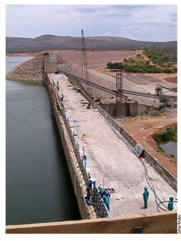
of the dam was extended from 770 m to 1 150 m and the right rollcrete flank from 215 m to 270 m. The smooth spillway was raised by placing a 5 m-wide stepped layer of rollcrete against the downstream face. Rollcrete
