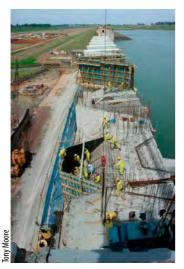
supply water to both towns as well as for agricultural use. The uMgeni Government Water Scheme was approved by Parliament in 1961, and that same year the DWA construction team moved onto site. The original dam wall was of the composite type, having a mass gravity concrete overspill section with earth flank walls. At the height of construction, more than 600 people laboured on the project. The dam was eventually completed in 1964.
