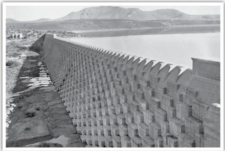
back stepped instead of battered. About 149 088 m<sup>3</sup> of concrete was cast in the construction of the dam wall which has a crest length of 500 m and a crest width of 3 m. The spillway is 303 m long.
