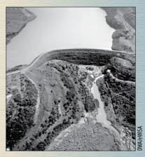
Bridle Drift Dam from the air. The original earth and rockfill dam wall was 518 m long at the crest and 52 m high.
