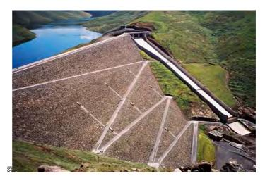
Left: Around 100 000 m<sup>3</sup> of concrete and 7,2 million m<sup>3</sup> of rockfill went into the Mohale Dam wall.
