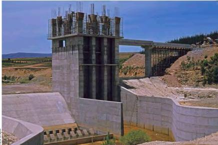
Left: The Charmaine wall structure under construction in December 1976. The wall, which houses the Charmaine intake and outlet is situated inside the basin of the Theewaterskloof Dam.
