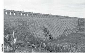
Left: Nqweba Dam (formerly known as Van Rynevelds Pass Dam) is a mass concrete wall of gravity section.
