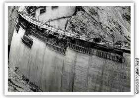
expensive. This was the first dam of its kind to be constructed in South Africa. The DWA project team developed a mathematical mesh model to obtain the optimal shape of the dam and ensure minimum bending within the shell. Solid model laboratory tests were also undertaken – another 'first' for the department.
