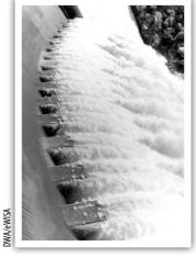
**Top left:** Blyderivierspoort Dam is a concrete gravity arch dam. It was one of the first dams in the country where computers were used in the design calculations.
