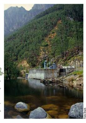
of the side-channel type and the chute ends in a stilling basin.
