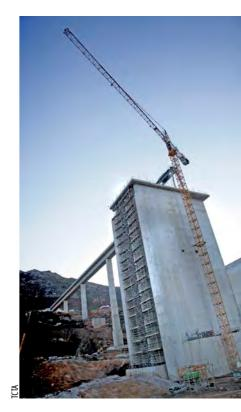
The south section of the Berg River Dam intake tower is an open vertical shaft (wet well) with multi-level gates for drawing water from the dam for high flows/floods (up to 200 m<sup>3</sup>/s) as required by the Ecological Reserve.
