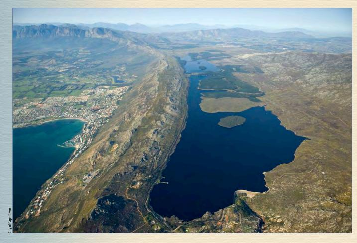
**City Engineer DE Lloyed-Davis the** Steenbras Dam, 50 km outside the city, was at last constructed in 1921. Built on the slopes of the Hottentots-Holland mountains, the first Steenbras Dam was a modest masonry structure (by today's standards) in the manner of the Table Mountain dams, and impounded 27 000 m<sup>3</sup> behind an 8 m-high wall. A pipeline of 76 km transported the water to the Greater Cape Town. Construction of the dam was
