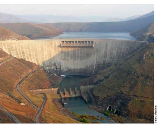
About 2,3 million m<sup>3</sup> of concrete was used to construct the 185 m-high Katse Dam wall. flood overflow of 6 250 m<sup>3</sup>/s. This water flows into a plunge pool, created by a 32 m high tailpond dam with a shaped ogee weir, which is situated 100 m from the base of the dam wall. The crest is 9 m wide, incorporating a roadway.
