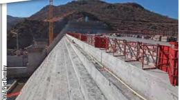
The De Hoop Dam spillway as it stood at August 2011. The special rollcrete mix negated the need for skin concrete.
