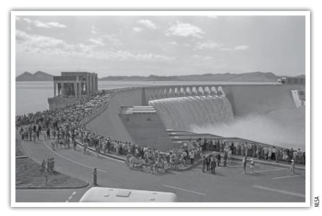
openings are situated in the water intake sections, three on each bank, symmetrically positioned, and there are six large concrete channels or chutes – three on each side and a concrete apron beneath the overspill to prevent the falling water from eroding the rock at the base of the dam. Under normal maximum flood conditions 8 000 m<sup>3</sup>/s of water can be discharged. This is in addition to the 8 100 m<sup>3</sup>/s of water which can be discharged through the chute spillways.
