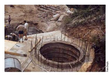
Left: The Banhoek shaft under construction in 1979. The shaft is 162 m deep and 1,8 m in diameter.
