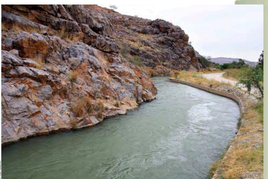
Although the dam had an initial storage capacity of 40 million m<sup>3</sup>, this has been halved through sedimentation. The sediment sluices have been closed permanently and the structure is now effectively a concrete weir which supplies water into the canal on the left bank. Today, the Buchuberg canal supplies water to 7 560 ha of irrigated area, most of which is used for field crops and a small portion of fodder crops.
