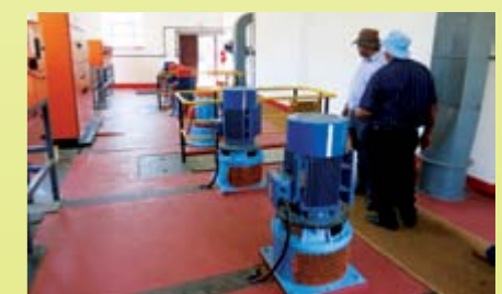
Ronald Brown and Cedric Morkel discuss on-site issues.
