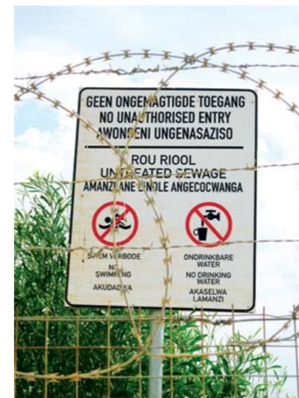
Fencing and onsite security are a high priority on the plants.
