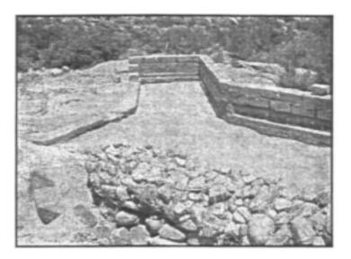
Plate 7 The filter ready for operation, showing the new gabion, the new wall and filtered river sand covering the surface of the filter.
