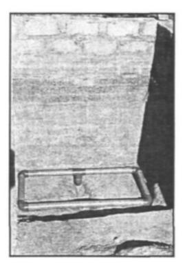
Plate 5 Slotted PVC filter pipe at base of the sand filter. This is surrounded by coarse gravel (5 - 10 mm diameter), which is covered by 16/40 pool filter sand to 10 cm above the gravel, and then covered with 2mm sieved river sand to the top of the filter.
