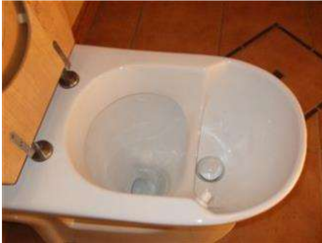
Figure 43 Dubbletten flush UD (left) and A dry composting toilet manufactured by Solazone (right)
