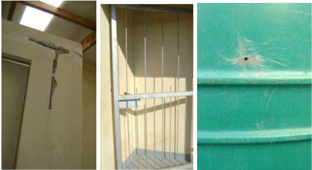
Figure 16 A damaged door frame, inadequate security gate and punctured Jojo tank
