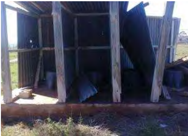
Figure 7 Girls' toilets damaged by winds (left) and boys' toilets without a superstructure at Lower Qutsa
