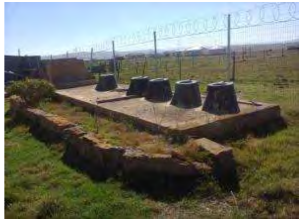
Figure 7 Girls' toilets damaged by winds (left) and boys' toilets without a superstructure at Lower Qutsa
