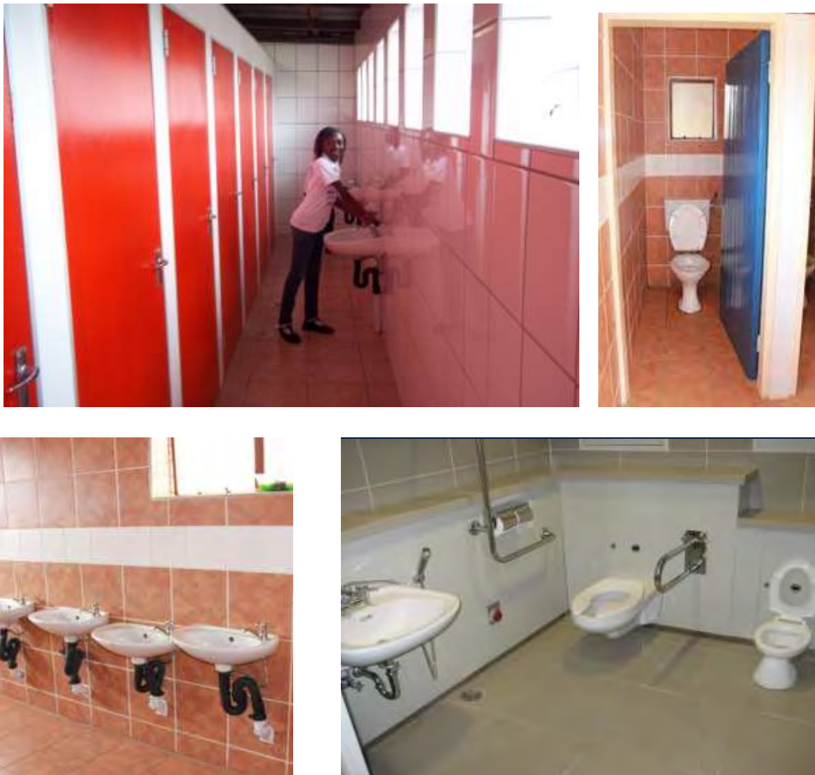
Figure 24 School toilets renovated by SAWASA (Source: Trevor Mulaudzi)
