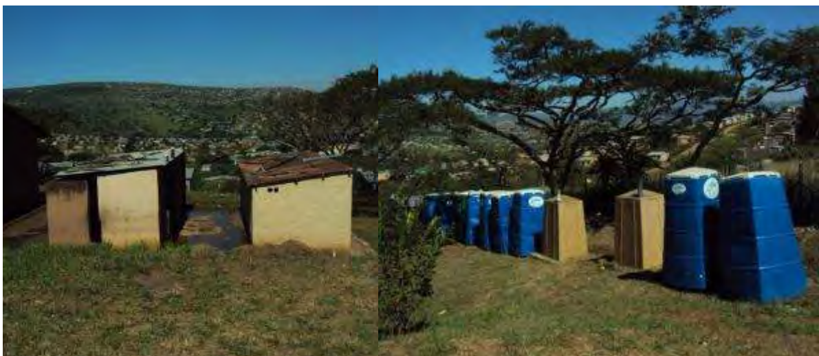
Figure 14 Full pit latrines (left) and bucket toilets (right) at Mumzo High School. The two beige structures (centre right) cover functioning pit latrines.
