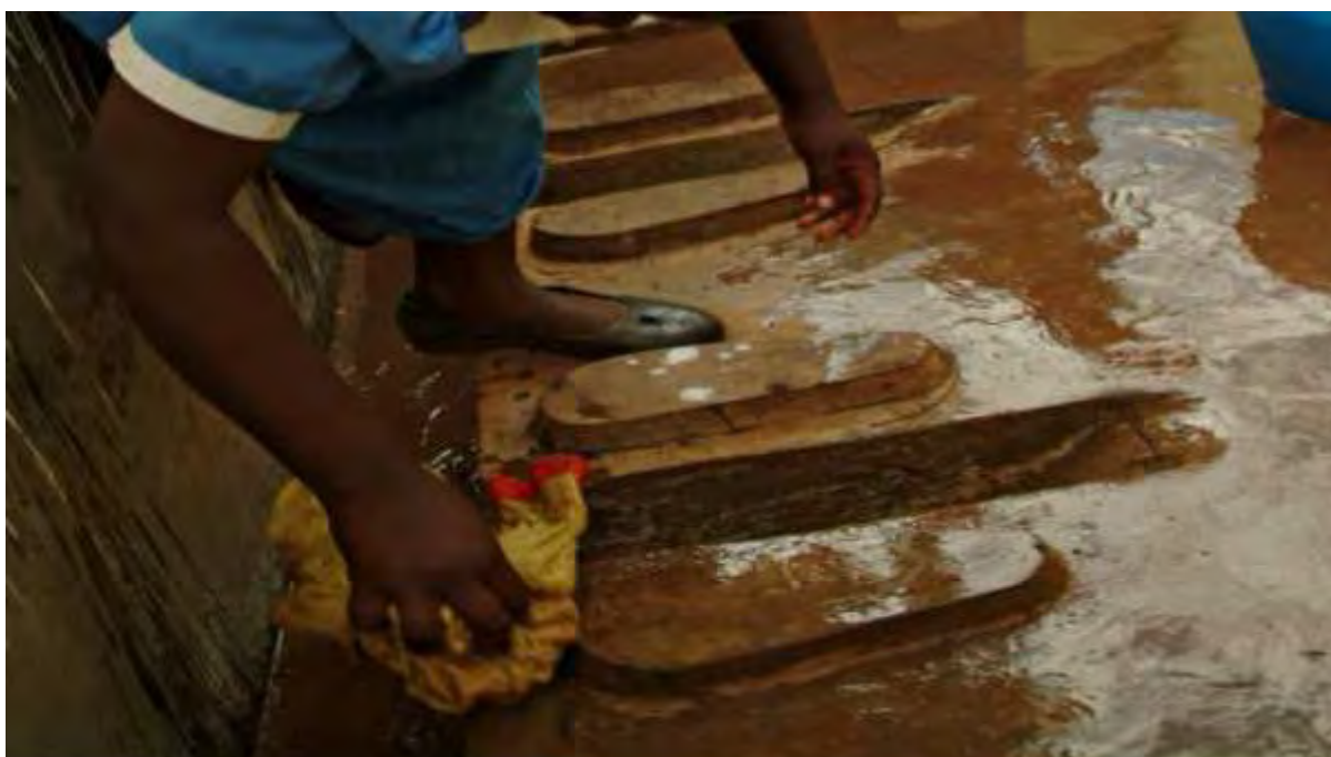
Figure 33 A female urinal design used in schools in Malawi 21
