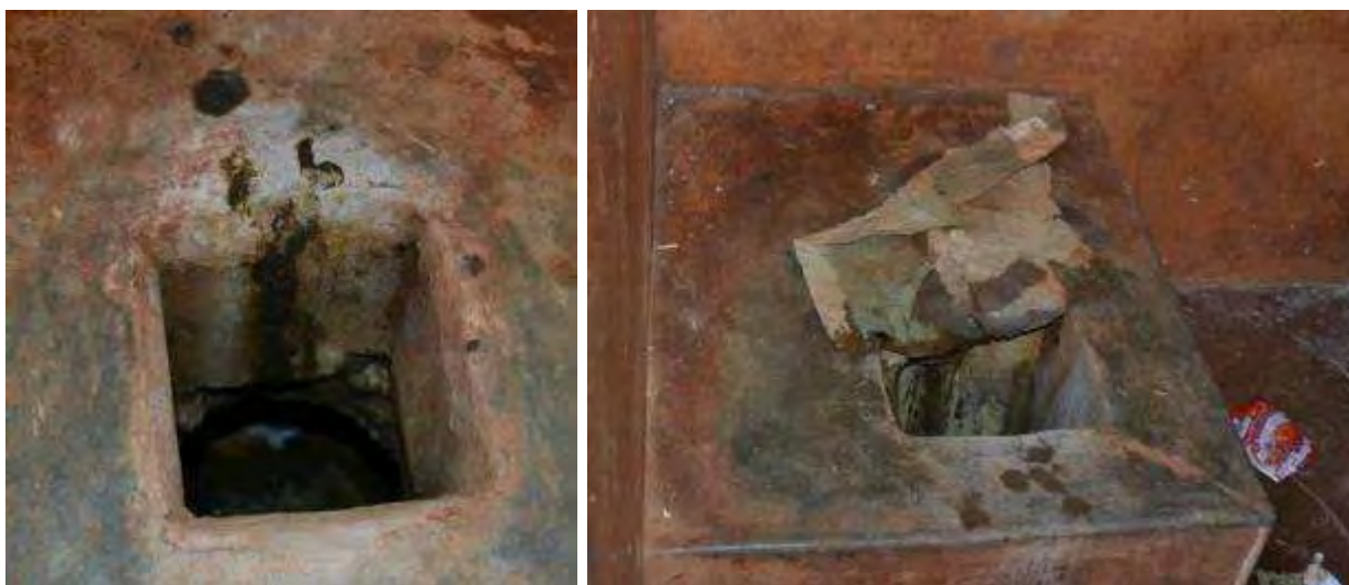
Figure 18 Toilets at Lutandale Primary School
