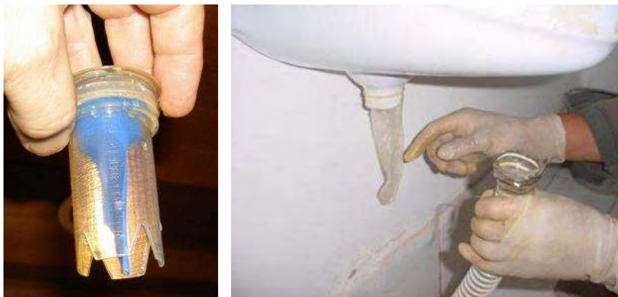
Figure 35 EcoSmellStop (ESS) from Addicom (right); a condom adapted as a water seal (right)
