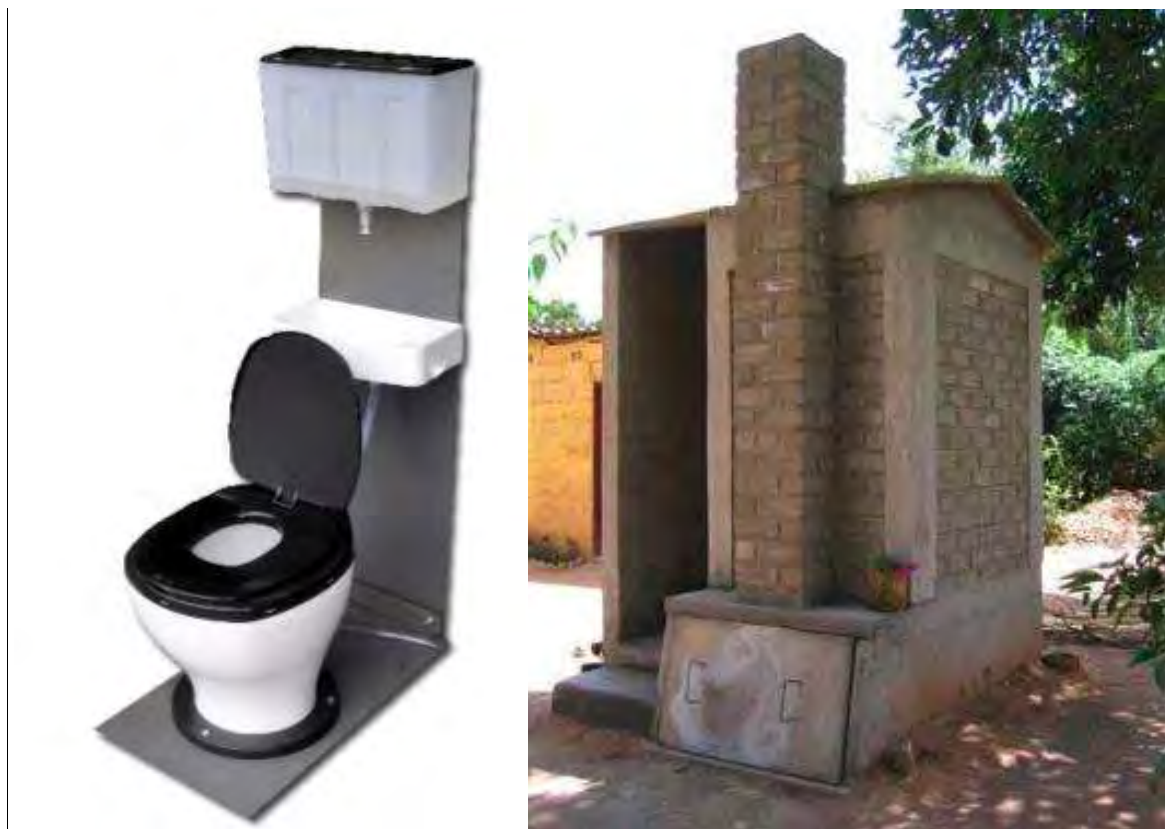
Figure 42 Left: UD flush toilet (Envirosan); right: dry UD toilet used by eThekwin Municipality
