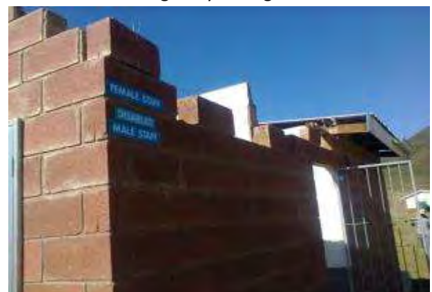
Figure 6 Roofless teachers' toilets at Lower Qutsa
