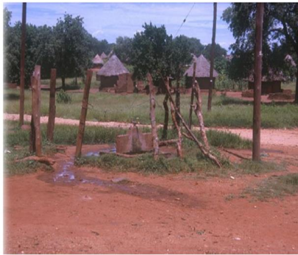
Piped water supply
