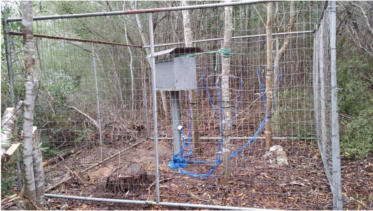
Figure 8.2: Sap flow monitoring system installed on the hillslope
