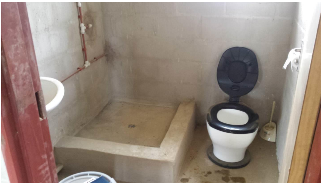
Figure 12: A view of a Pour Flush toilet in a bath room in one of the Oakford houses.
