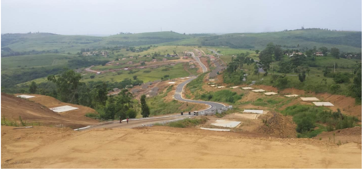
Figure 4: Housing under construction at Oakford.
