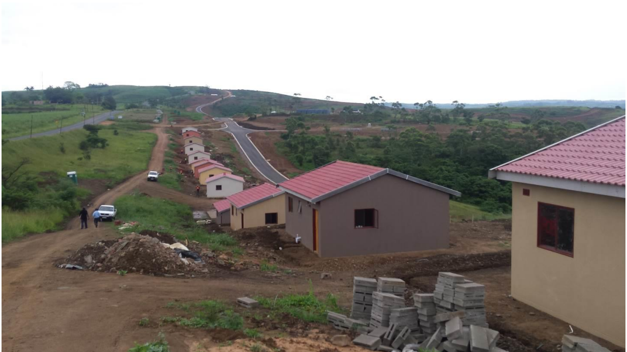
Figure 5: A view of the first set of houses nearing completion.
