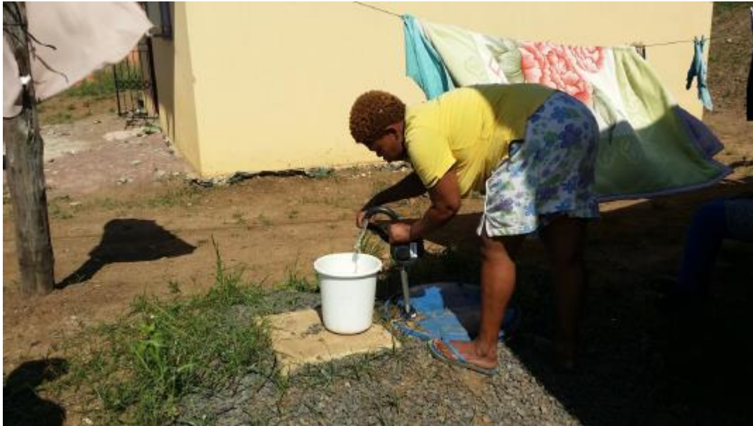
Figure 13. The greywater collection tank with handpump fitted for extraction of flushing water. The water is filtered through sand and geofabric before it enters the collection drum.
