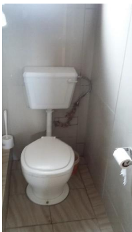
Figure 14: Pour Flush system retrofitted with cistern by the eThekweni Housing Department. The cistern installation was in response to pressure brought to bear on them by community representatives who did not fully understand the cistern-less Pour Flush system (to reduce water leaks). The homeowner tiled the bathroom which shows a sense of ownership.
