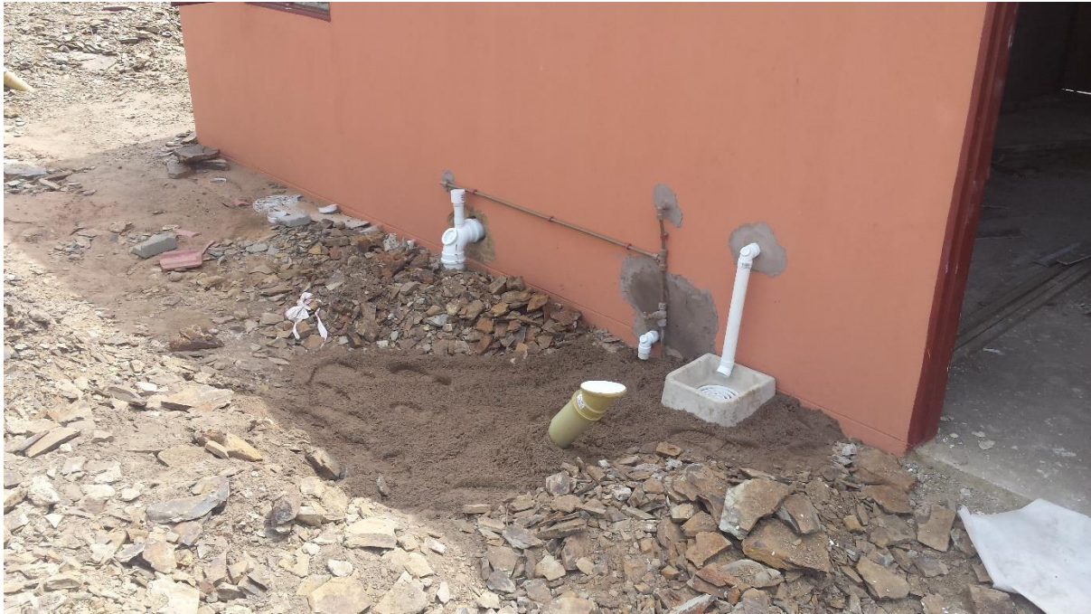
Figure 6: Ground conditions at some sites have been particularly difficult.
