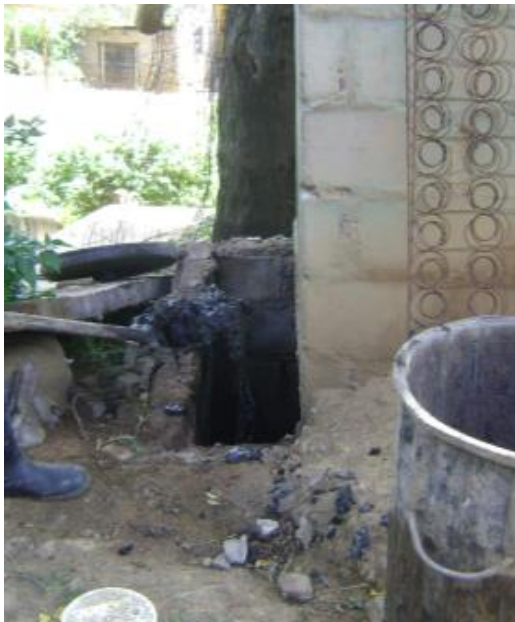
Figure 26: At these two sites sludge can be seen contaminating the lip of the pit and the area between the pit and the bin. There was no provision made to protect the earth between the pit and the bin.
