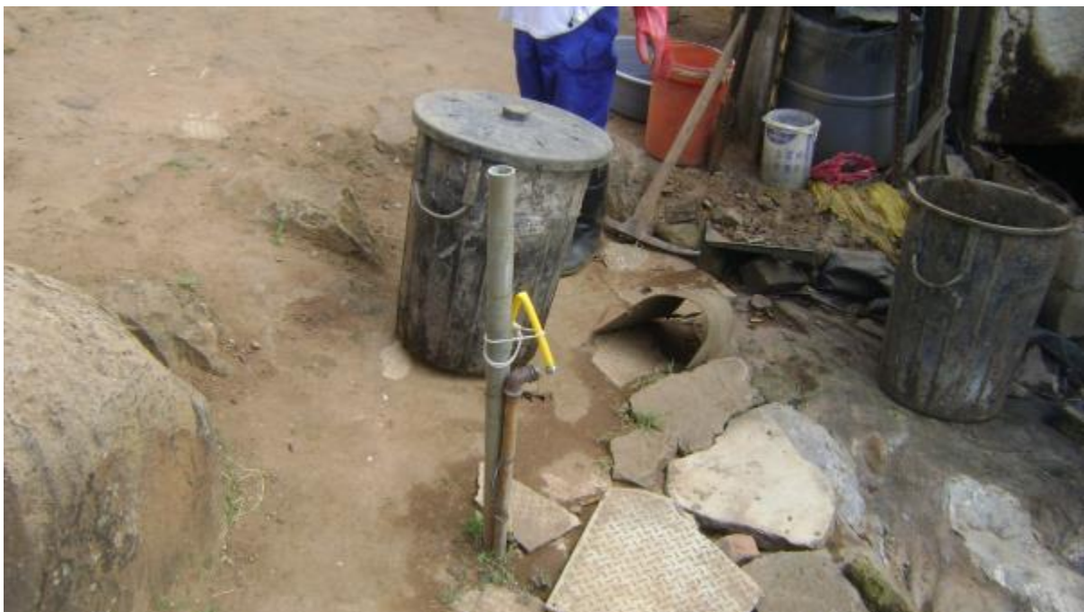
Figure 17: At this site workers worked amongst household objects and building rubble, risking greater contamination of the site.
