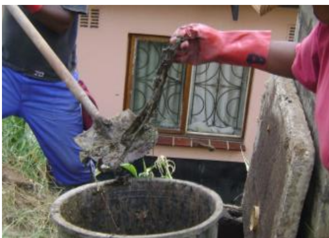
Figure 14: A worker handles trash in the sludge directly with her hands, heavily soiling her gloves.
