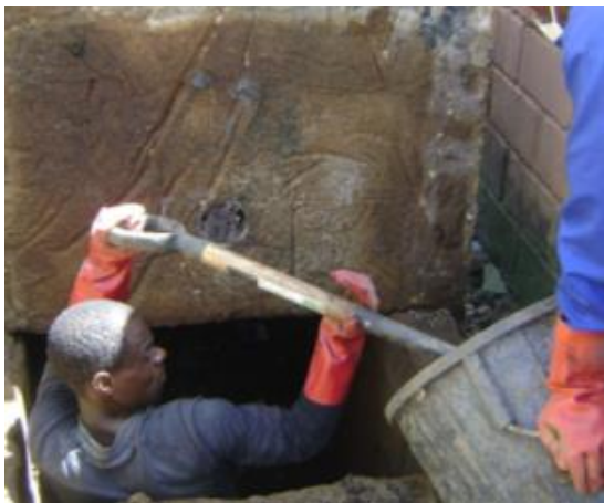
Figure 24: These workers have entered the pit without a mask or protective jacket, putting themselves at unnecessary risk of infection in order to more easily remove the sludge. When they climb out of the pit their boots will track sludge around the household environment, into the vehicle and into their home, putting others at risk of infection as well.
