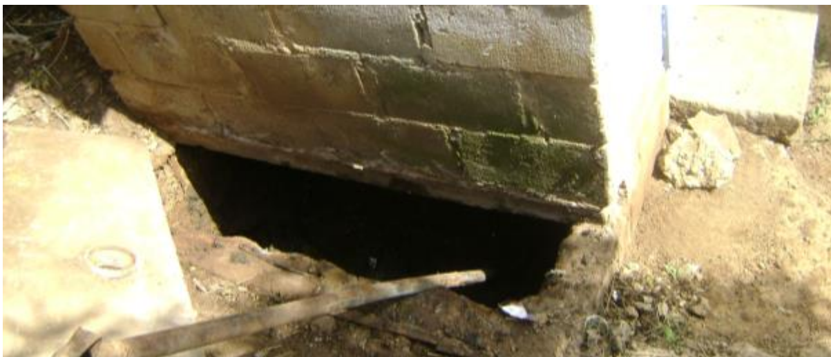
Figure 22: Access to the pit was sometimes very limited.
