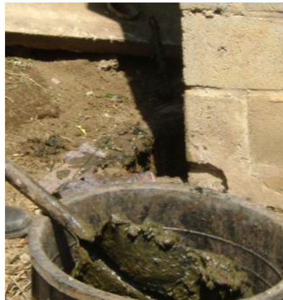
Figure 26: At these two sites sludge can be seen contaminating the lip of the pit and the area between the pit and the bin. There was no provision made to protect the earth between the pit and the bin.
