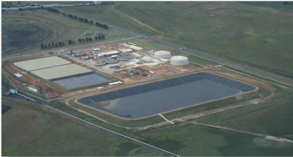
Figure 3.2: Aerial view of Emalahleni water reclamation plant in Mpumalanga (Source: http://www.projectlink.co.za/portfolio-item/project-water-treatment-plant/ )
