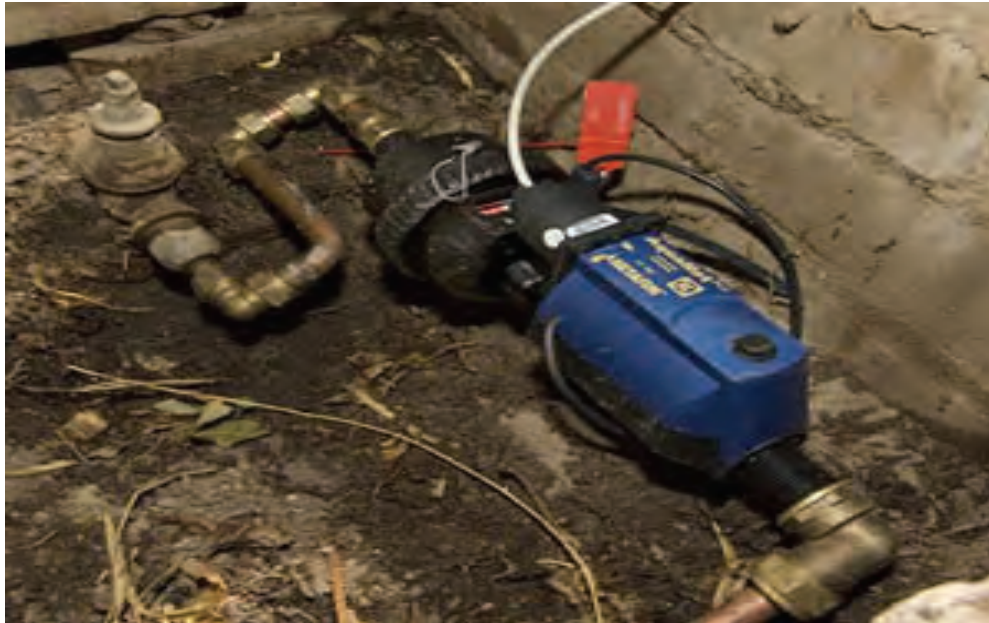
Figure 21 Water Management Device/ Flow Limiter – eThekweni
