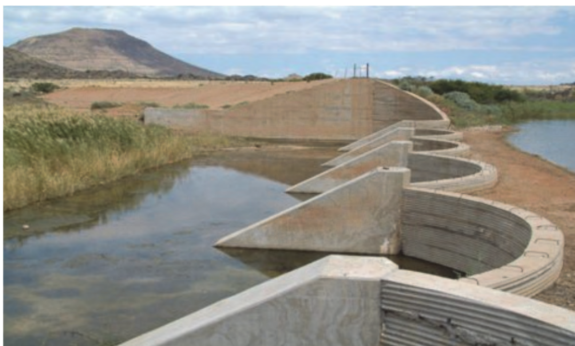
Figure 5.5 Old weir at Murraysburg (Source: S. Theron, personal communication)
