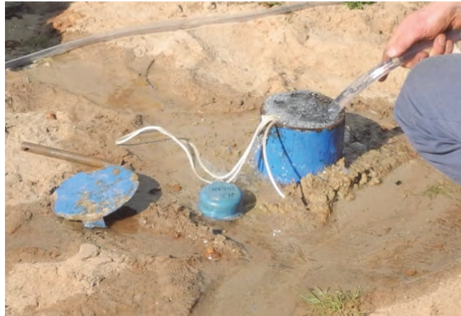
Figure 46: The project team struggling to get the injected ozonated water into the aquifer due to the bubbling and overflow from the injection well-point
