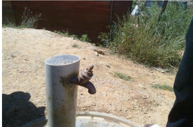
Figure 8: A broken tap in Kayamandi
