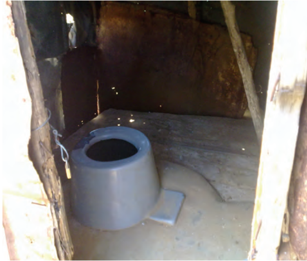
Figure 4: Pit latrine in Shembe
