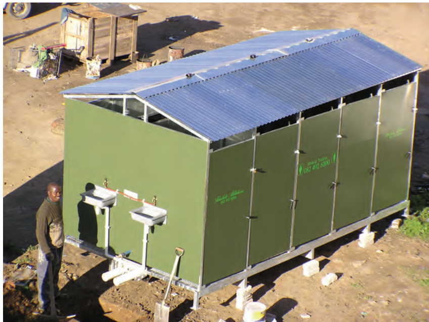
Figure 8: View of the installation of the Kayaloo unit
