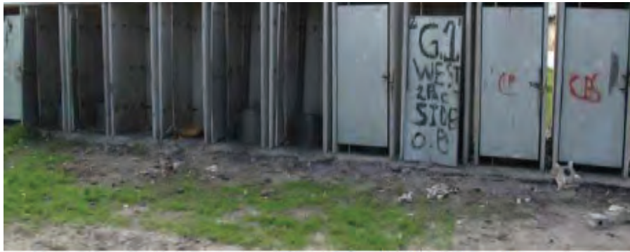
Figure 5: View of container toilets
