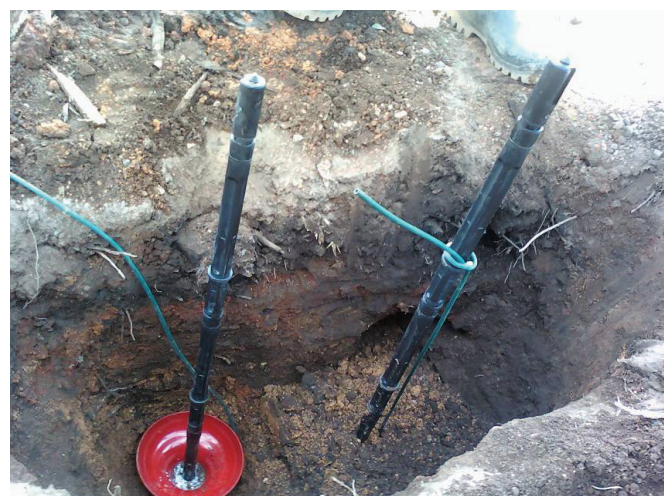
Figure 6.14 Installation of a pair of wetting front detectors at depths of 400 mm depth (left) and 1 m (right)
