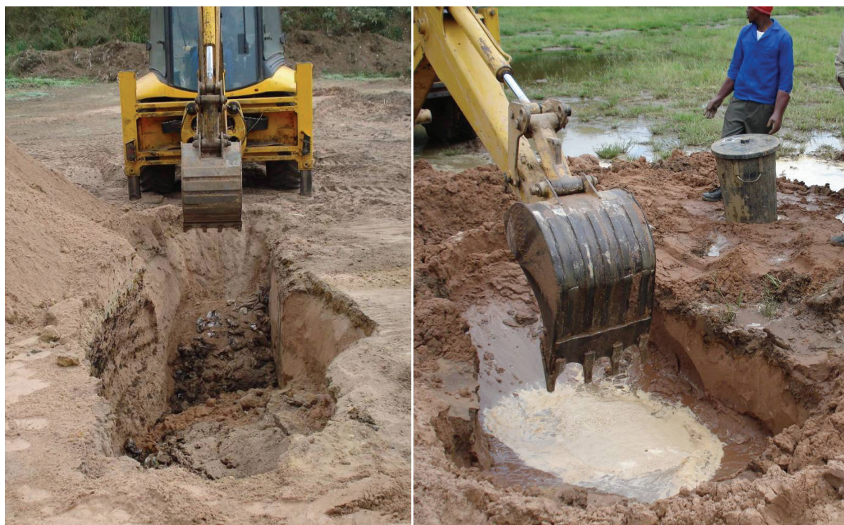
Figure 5.13 Variable conditions resulting in variable pit dimensions
