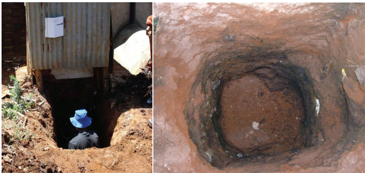
Figure 5.70 Manual excavation of a pit. Start of the sludge layer clearly visible 1.65 m below the surface.
