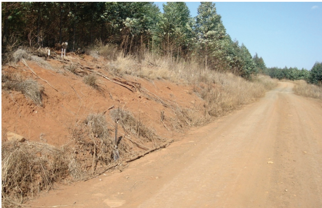
Figure 4.21. The cut slope of the road section studied. The soil is deep and well drained with no signs of exposed bedrock at the cutslope interface.
