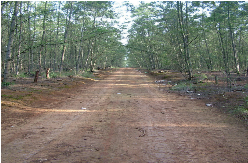
Figure 6.1. Road segment in a state of good condition.
