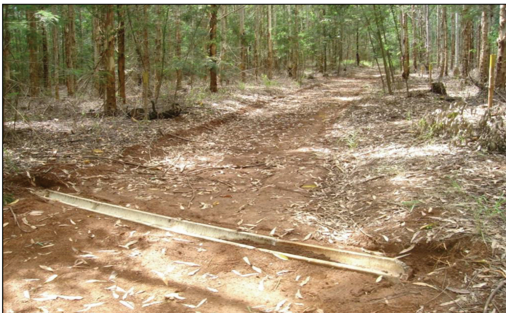
Figure 3.14. The completed gutter installed flush with the road surface.
