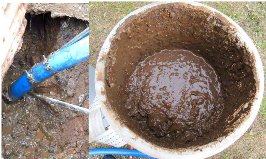
Figure 7.11 Emptying a pit with the eVac
