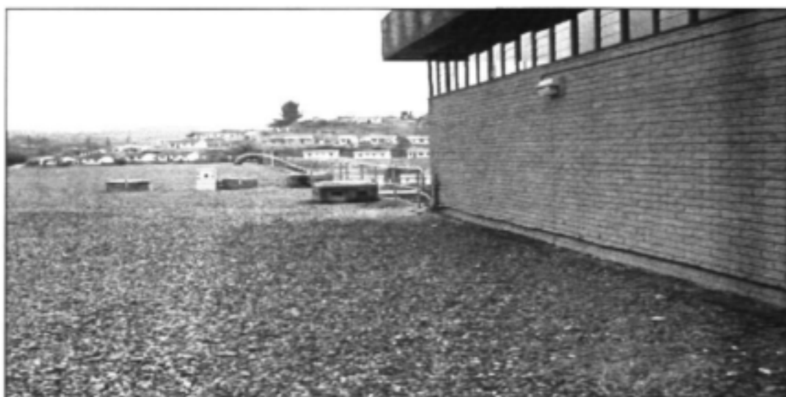
Figure 1.4 : View of the top of the reservoir
