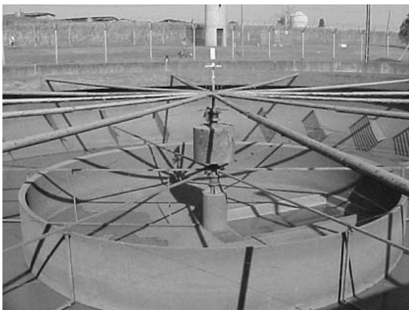
Figure 5.1: View of the central part of the clarifier before the upgrade.
