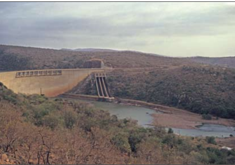
Pongolapoort Dam is a medium thin, double curvature arch dam with a gradual transition towards a gravity thrust block on the left flank.
