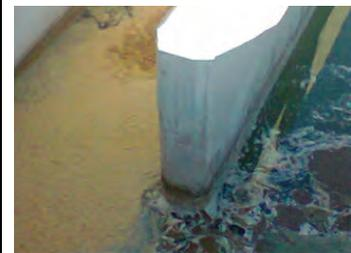
**Figure 5: Fat, blood and feathers collected in one of the corners of chlorine contact tank**
