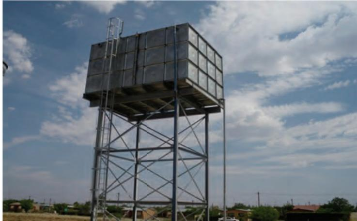
**Figure 7: Storage tank with treated wastewater for distribution to the connected houses**
