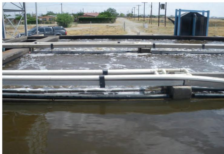
**Figure 6: Tokoloko – Close circuit wastewater treatment tank divide into three compartments of equal volume**
