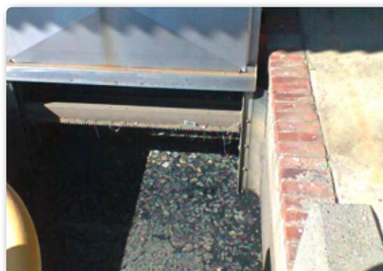
*Figure 2: Bloody wastewater turning septic in one of the inlet screens due to blockage caused by "thick" clots of blood in the wastewater*
