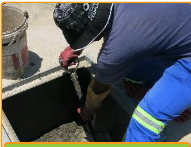
Weekly maintenance work performed by municipality workers.
